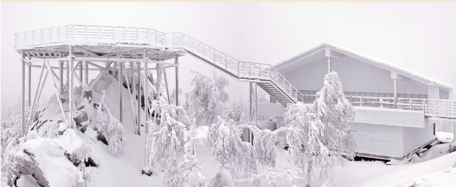
A fitness and health complex of the mountain ski centre "White Mountain". Framework construction. Capacity of 350 tons. 2008. Photo of 2012.
